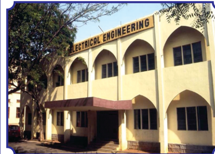
Department of Electrical Engineering
